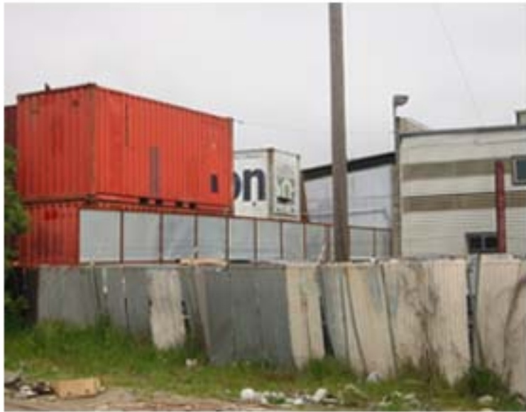
Looking at South wall over corner of 1017 Folger
