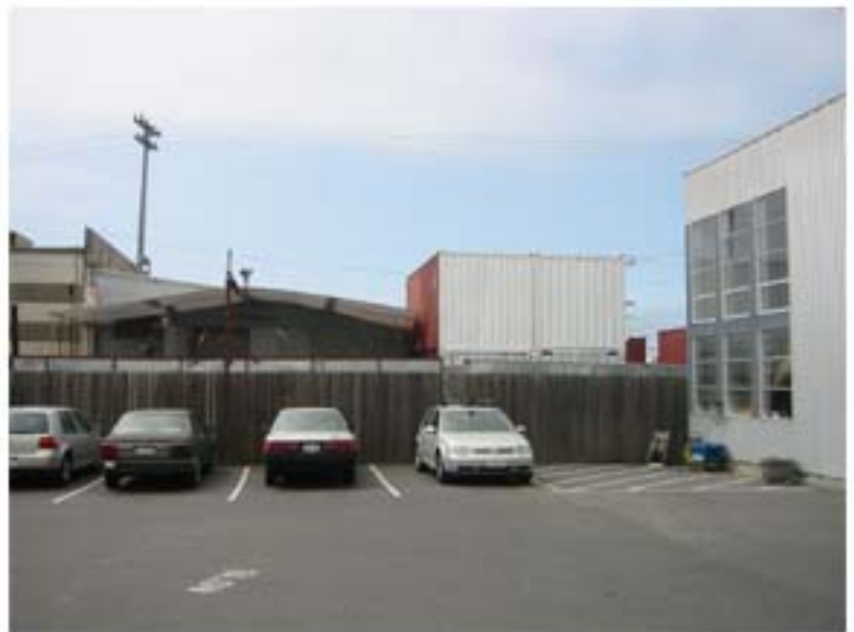
Looking at East wall from 1026 Murray Street
