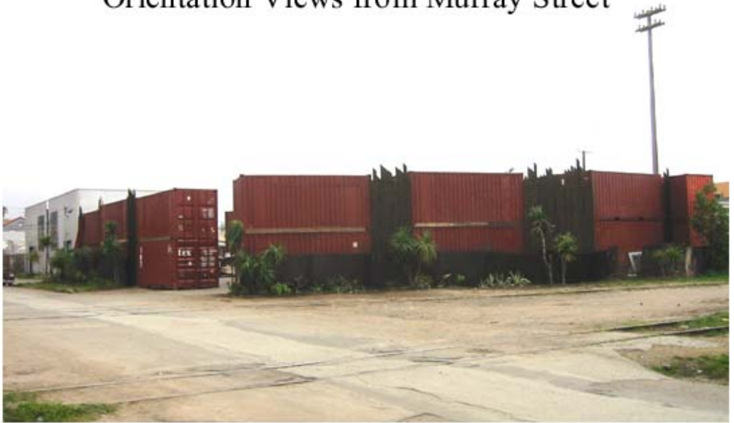
North and West outside walls of The Shipyard
