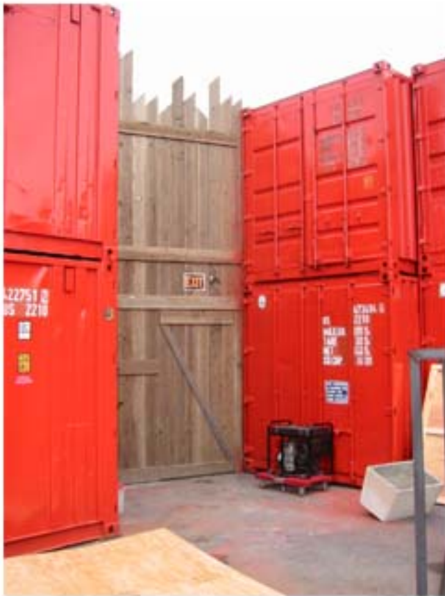
Detail View of Northeast corner
